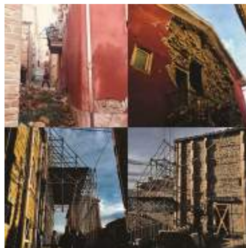
Fig. 1. Some photographs of the historical downtown of Gualdo, all red zone (photo credits: I. Passamani, 25/11/2017).
